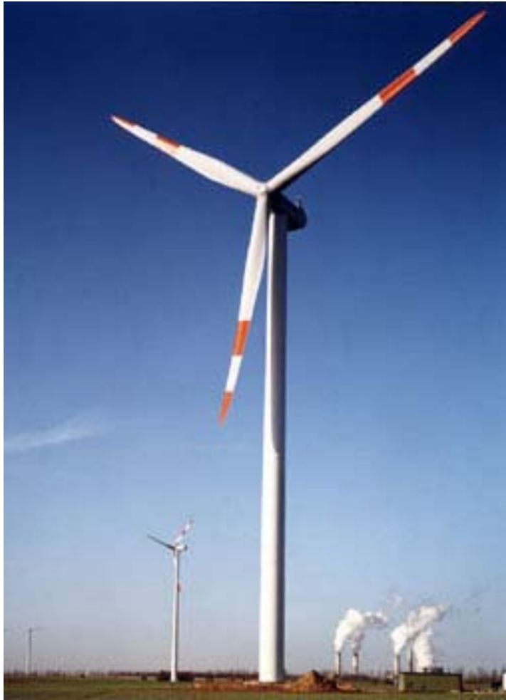
Prototype of 80 m tall Nordex 2,5 MW wind turbine located in Grevenbroich, Germany (Danish Wind Industry Association)
